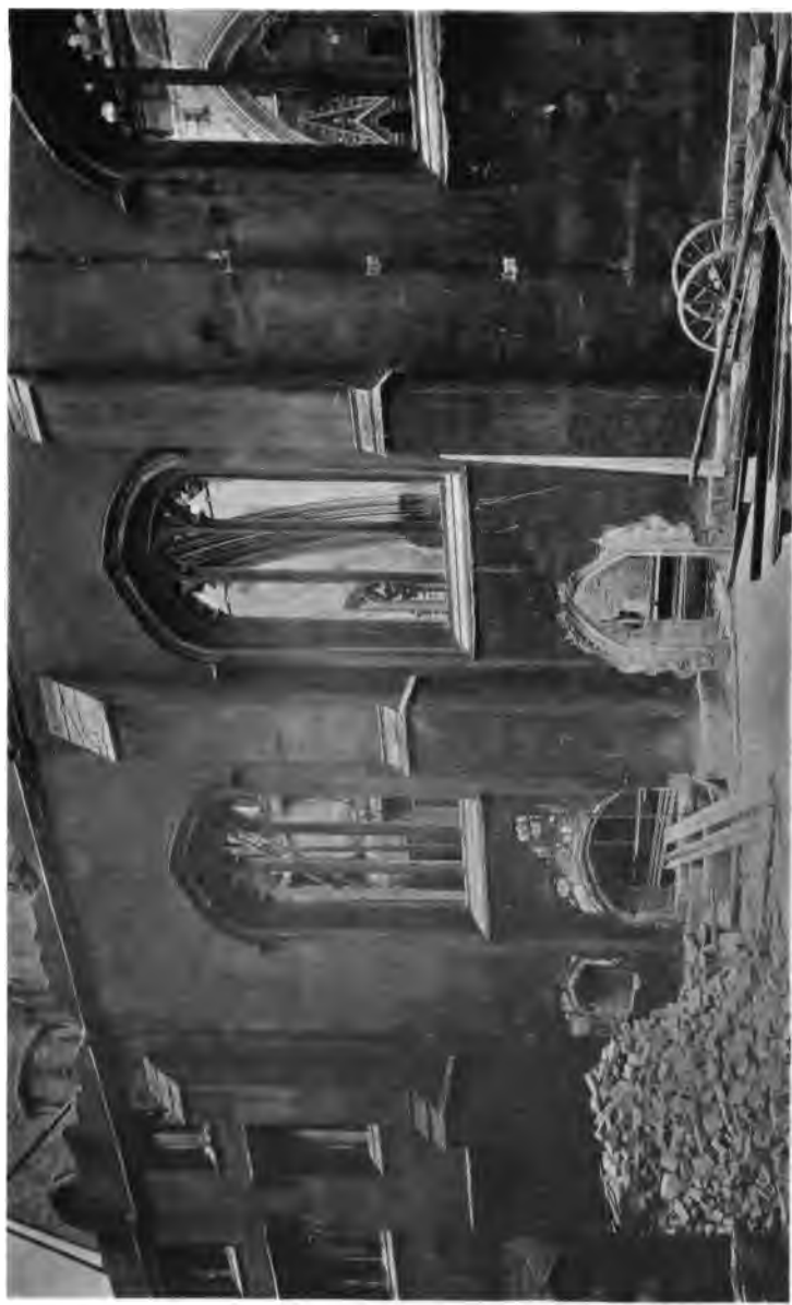
MIDDLE OF SOUTH SIDE. EXTERIOR.
